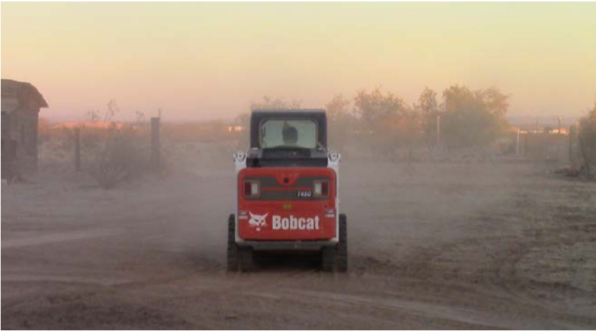
Grading the driveway with a track loader
