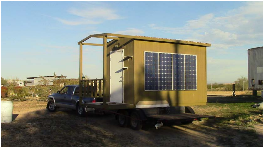
Final move for the solar hydrogen MicroDwell
